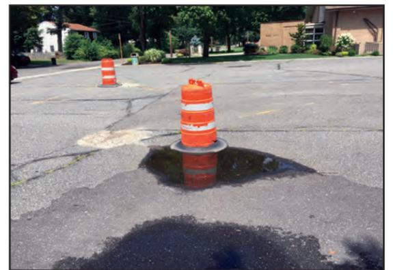
Our Parking lot suffers from severe cracking and improper drainage.
